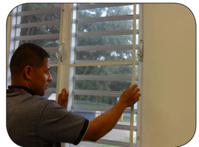
Install or repair window & door screens.
