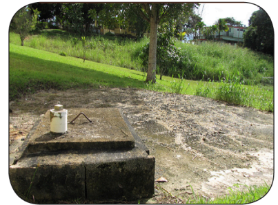
Keep septic tanks sealed.
